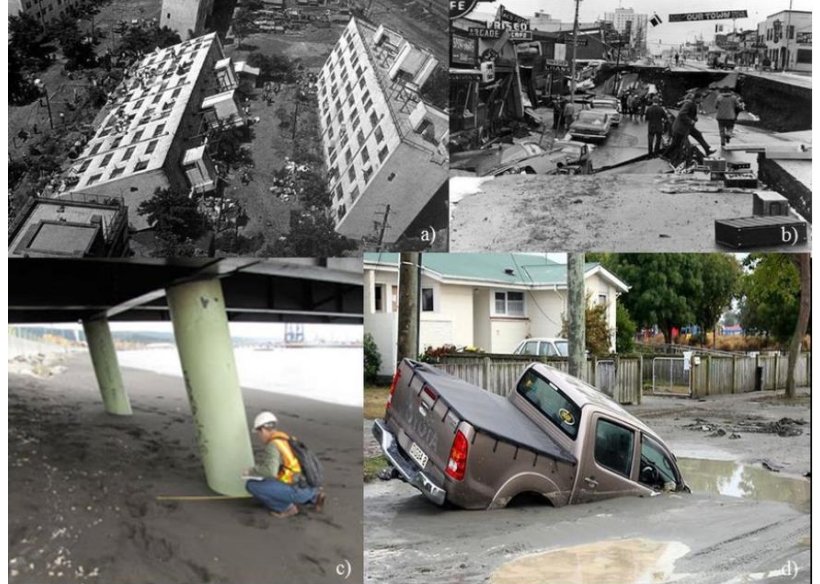
1. Liquefaction-induced damage observed in (a) Niigata, Japan 1964 (From http://civileggseminar.blogspot.d ), (b) Alaska, USA 1964 ( http://en.wikipedia.org ), (c) Maule, Chile 2010 (Provided by CGMI Consultants) and (d) Christchurch, New Zealand 2010 (From http://www.news.com.au ).
